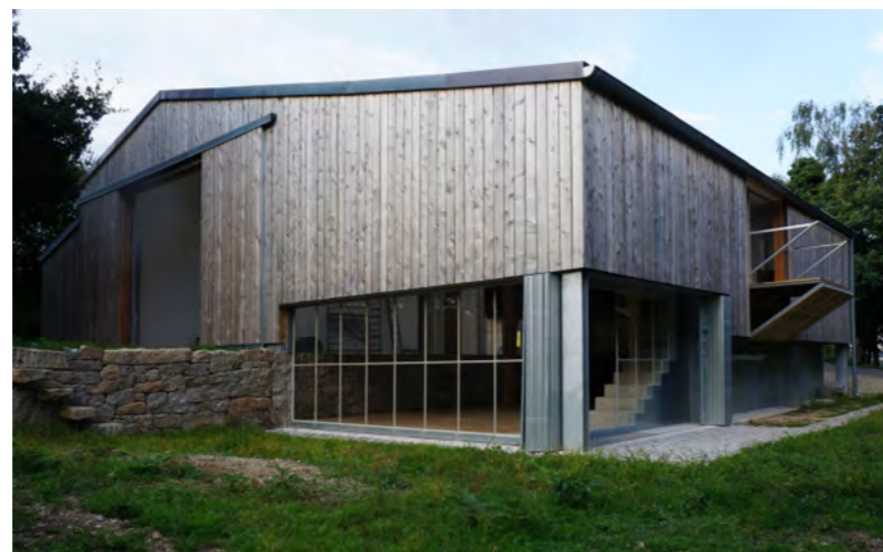
Timber barn with glazing and metal shutters
