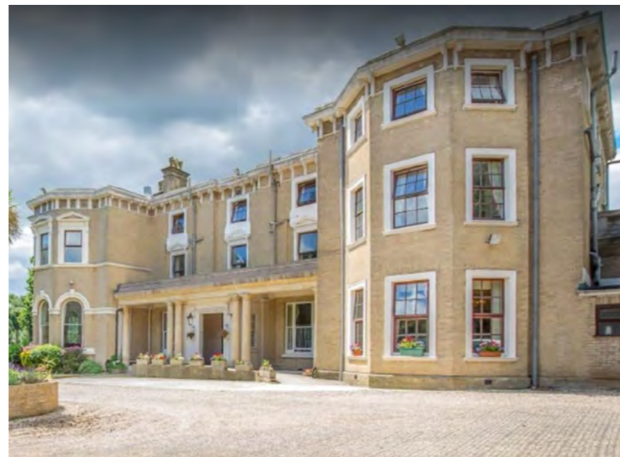
Coombe Lodge entrance (east elevation)
