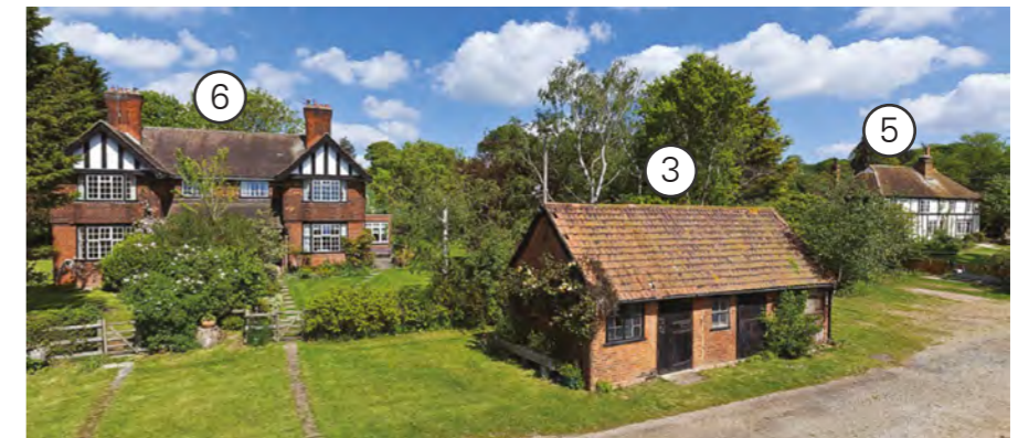
Buildings 3, 5 and 6 (image: Savills) - not part of application
