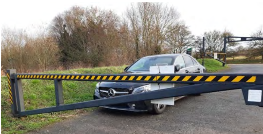
Vehicle security barrier
