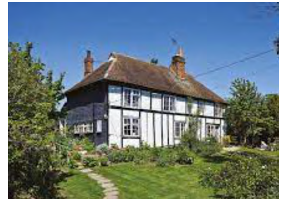
Grade II listed Farmhouse, Hole farm
