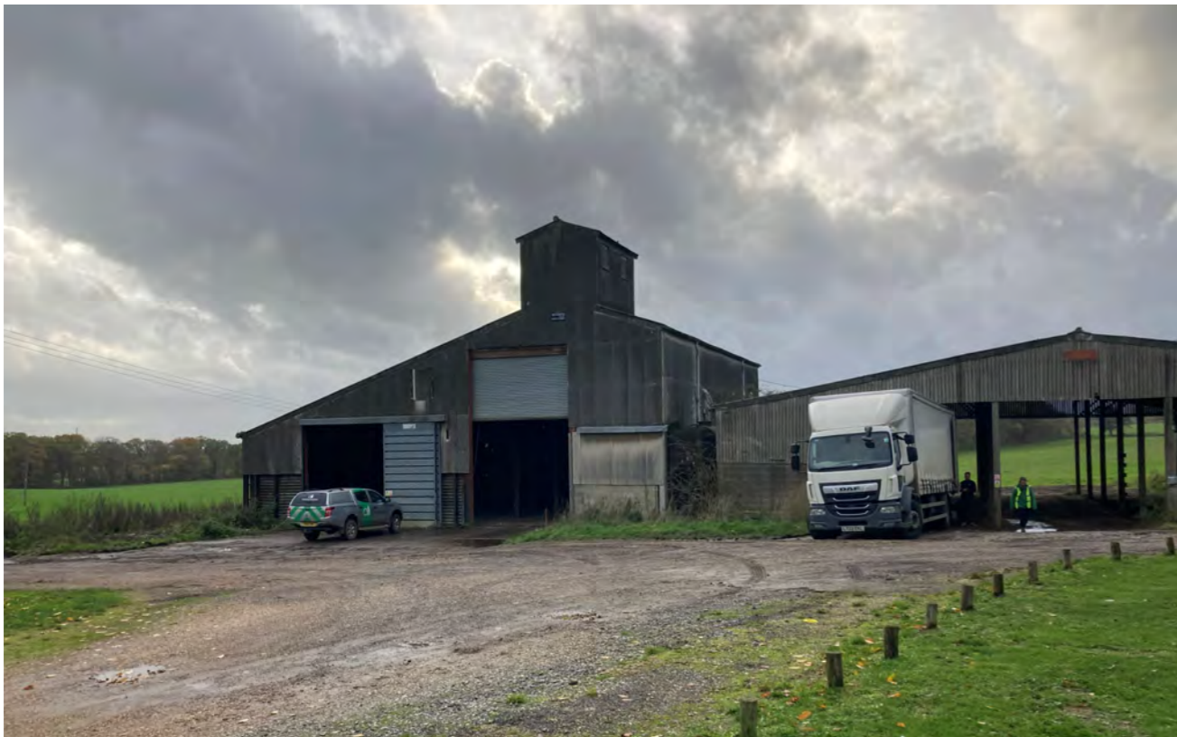
Building 1 left, Building 2 right
