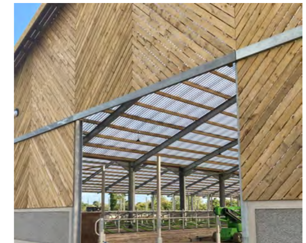
Herringbone pattern timber cladding
